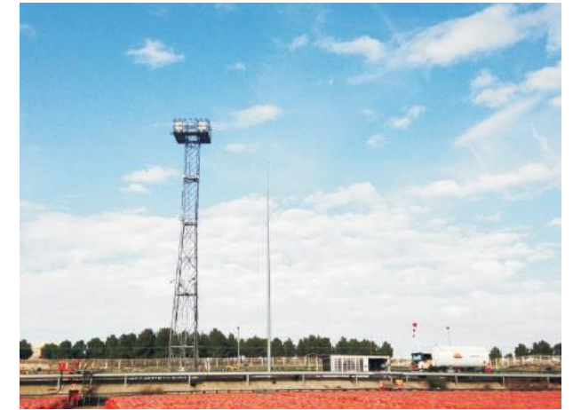
Gas holder Station ▲
